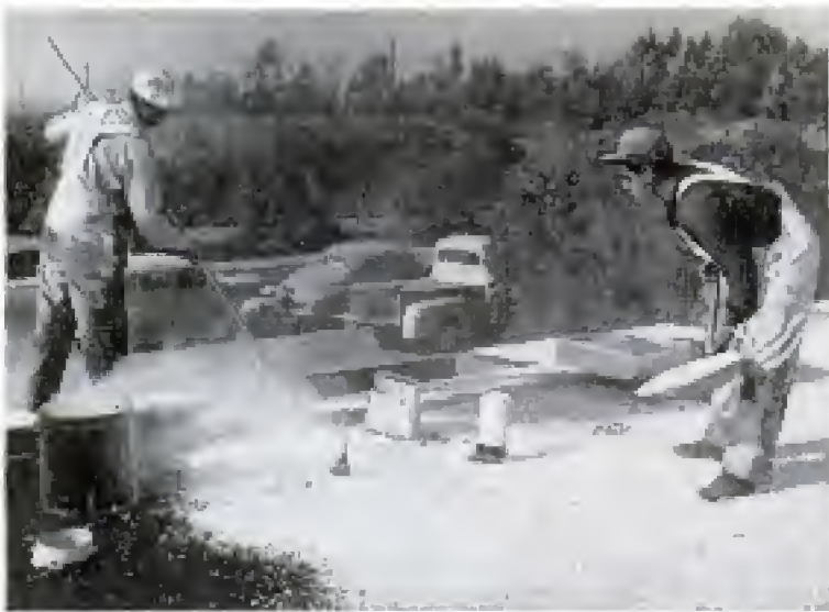
Roof panels in the slab-door house are topped by roofing paper, tar, insulating aluminum foil and final coat of crushed gravel
